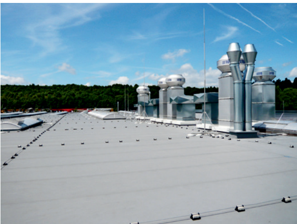
Schedetal SystemFlachdach in Stuttgart.
